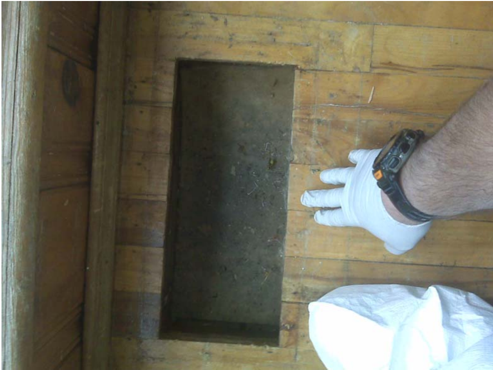
Photograph 1 Duct Interior Northeast Corner of Family Room
