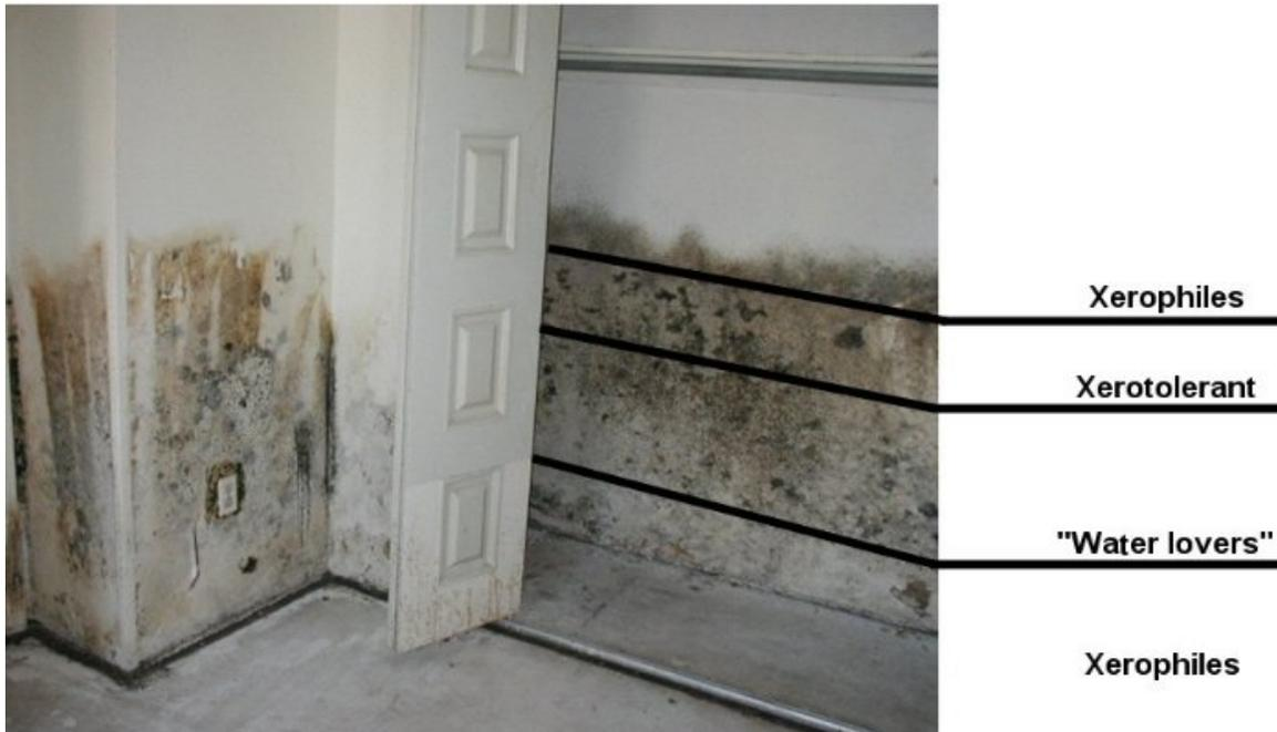
Moulds have “habits” and the habit speaks volumes to the inspector who will take the time out to listen. The habit can tell you why a mould is growing: is it due to condensation? Or thermal bridging? Or is it a water leak? Or a construction defect?
