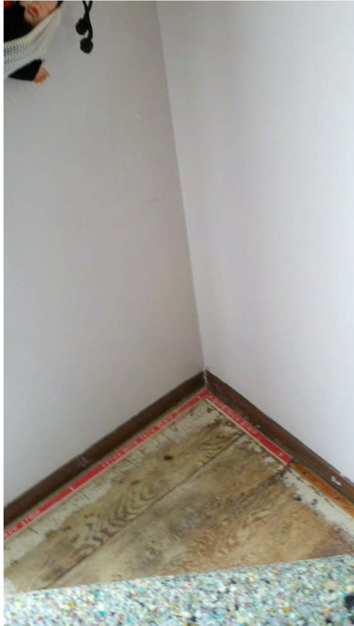
Photograph 2 Second Floor Bedroom Northwest Corner
